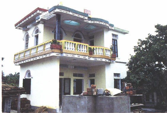
Photo 9 A new building under construction
